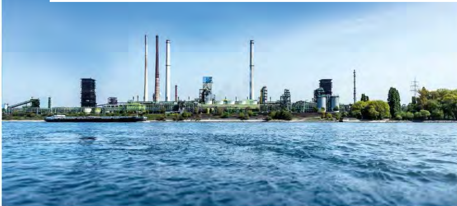
thyssenkrupp is accelerating the green transformation: Executive Board of thyssenkrupp AG releases capital resources for construction of Germany's largest direct reduction plant for low-CO 2 steel at the Duisburg site. Investments of more than two billion euros - subject to public funding - planned.
